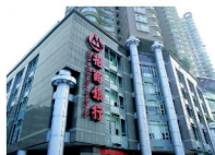
Construction Outer Wall
